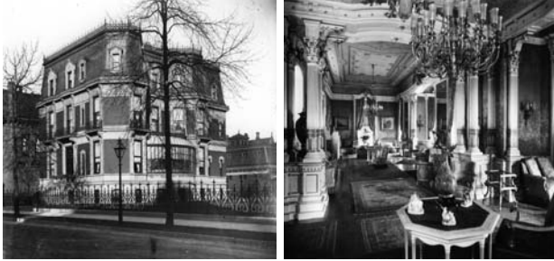
(Left) Field Mansion, 1905 South Prairie Avenue (Right) Pullman drawing room, 1729 South Prairie Avenue
