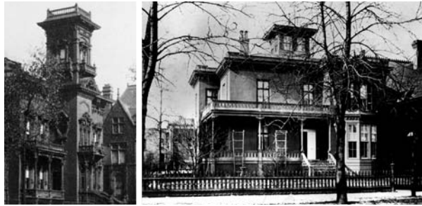
(Left) Thompson House, 1936 South Prairie Avenue (Right) Staples House, 1702 South Prairie Avenue
